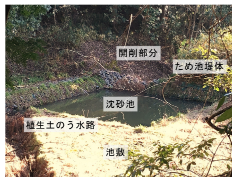
Fig.6 上流に沈砂池を設けた廃止事例 Abolition case of construct a settling basin upstream
