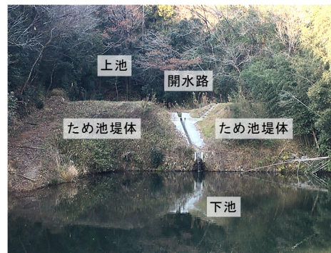
Fig.5 親子ため池での廃止事例 Abolition case in piled small earth dam for irrigation
